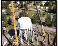
**Water Improvement Project- The** Water tower on Menser has finally been raised! The Water Tower now stands 53 feet taller, bringing the total height of the Water Tower to 153 feet!
